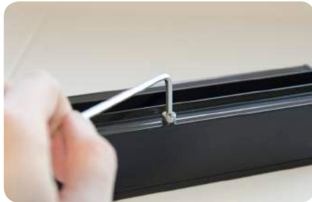
Unscrew side channels covers and profiles
