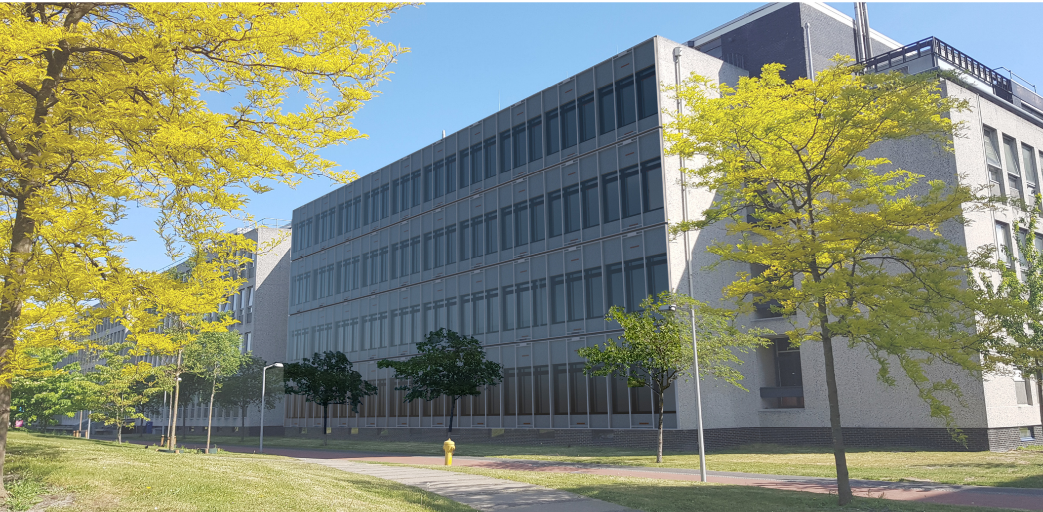
Figure 52: transparent PV-Trombe wall exterior view. Image by author.
