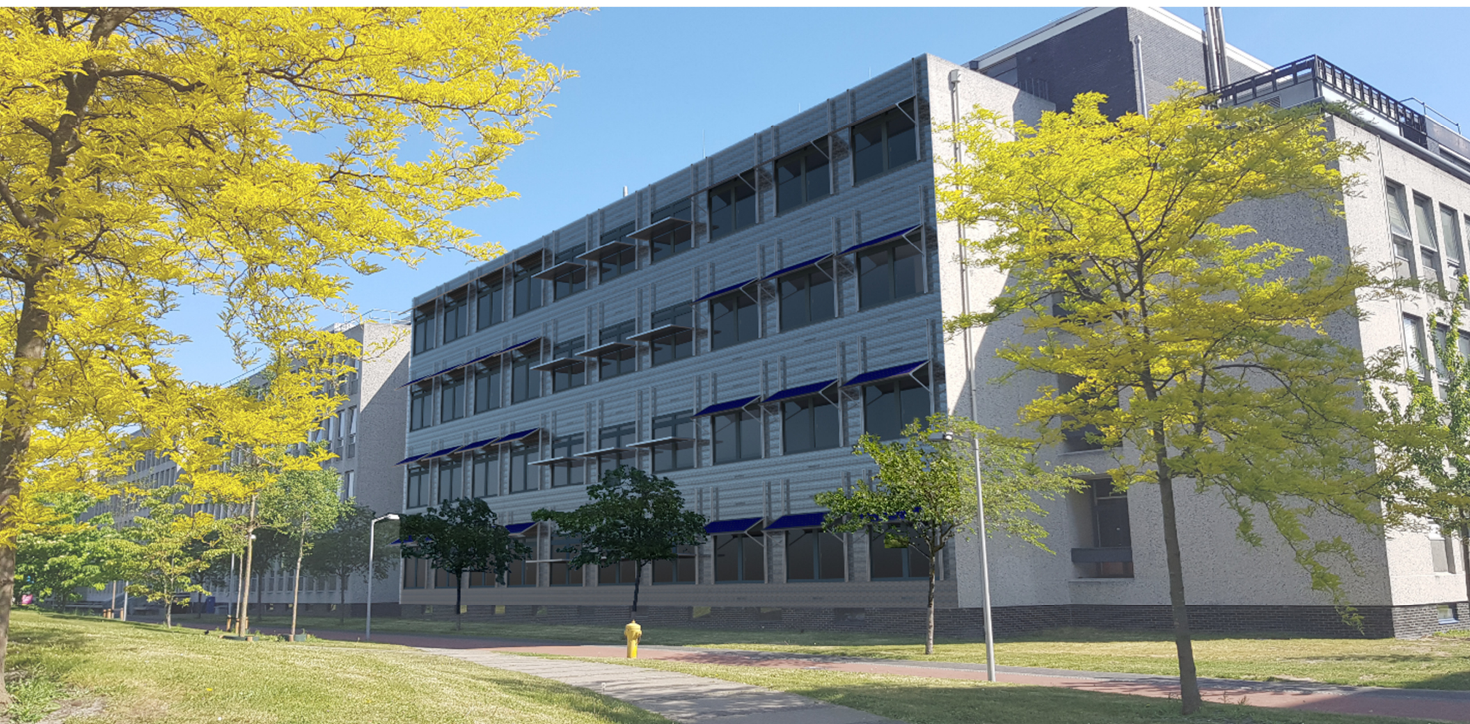
Figure 59: PCM Living wall exterior view. Image by author.
