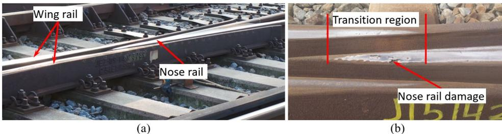
Figure 1.2. A 1:9 cast manganese steel crossing: (a) View of a wing rail and crossing nose rail; (b) Crossing nose rail damage in the transition region.
