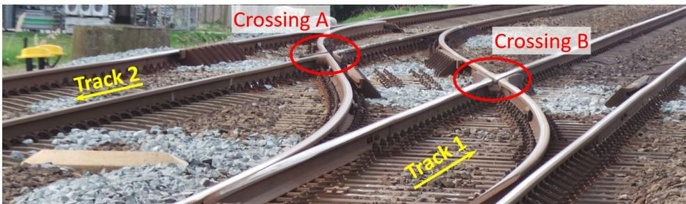
Figure 2.1. Typical crossover in the Dutch railway network.
