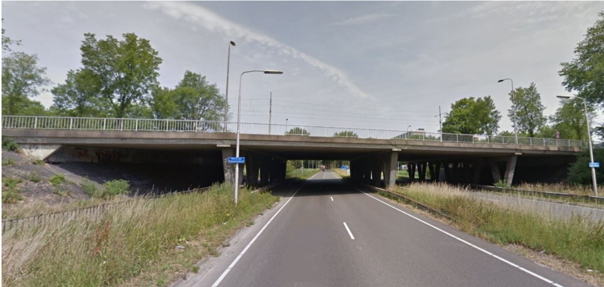
Figure 2.1: Example of a multiple span RC slab bridge, located in Delft constructed in the 1960s, from Google (nd).
