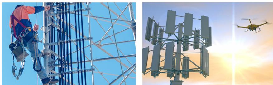
**Figure 1-1:** Manual inspection (left) can be replaced with a digital twin, captured using a remotely operated drone (right).
