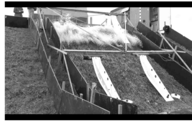
(b) Separation from the landside slope
