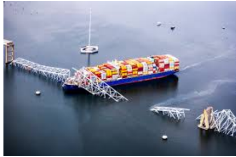
Figure 1.8: In 2024, a power failure on a container ship led to a complete loss of maneuverability, resulting in a crash that caused the Baltimore bridge to collapse. [18]"
