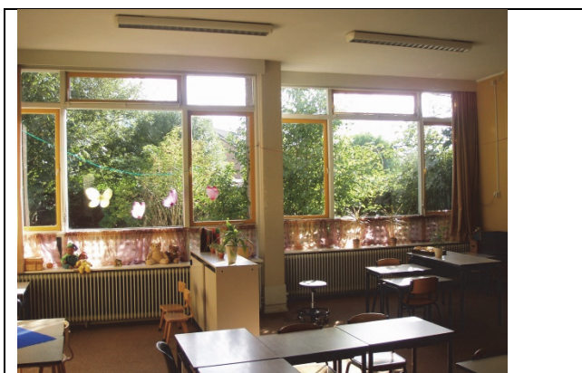
Figure 3.1.4: Example of a naturally ventilated school in Middelburg from around 1960. There are sufficient windows with different size and location and thermal mass that can be cooled down. Outside sunshade is available. The climate system was unchanged in 2006 when this picture was taken.
