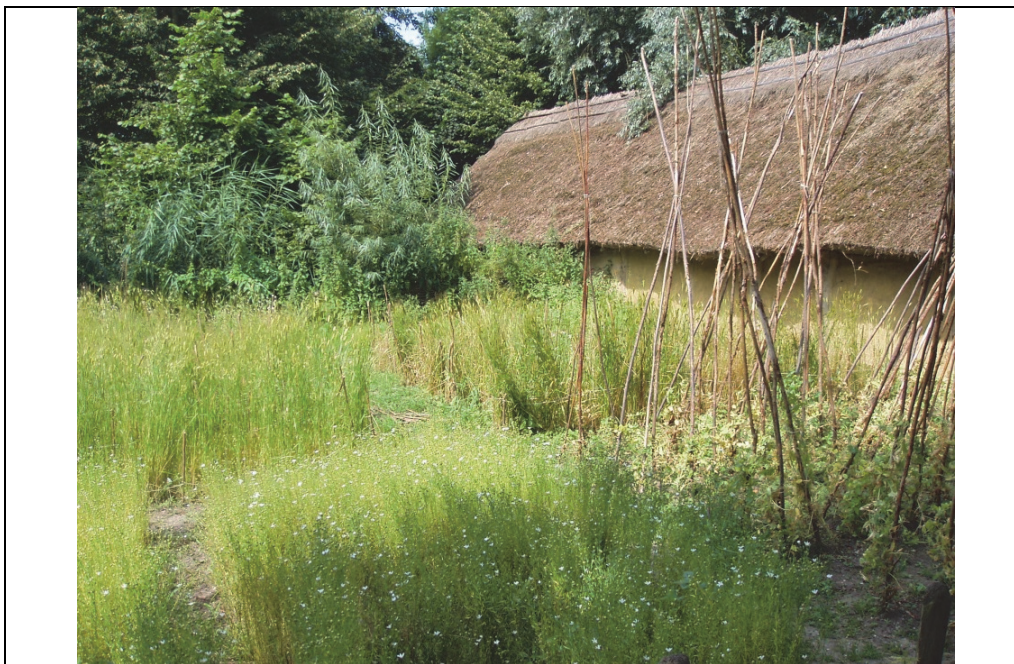
Figure 2.3.2: An aerodynamic shape, enough thermal mass, small windows and protecting trees are basic starting points for comfort in winter and summer. This was already known in the iron age. Of course, nowadays requirements are more complex and demanding, but basic starting points have not been changed. Archeon.
