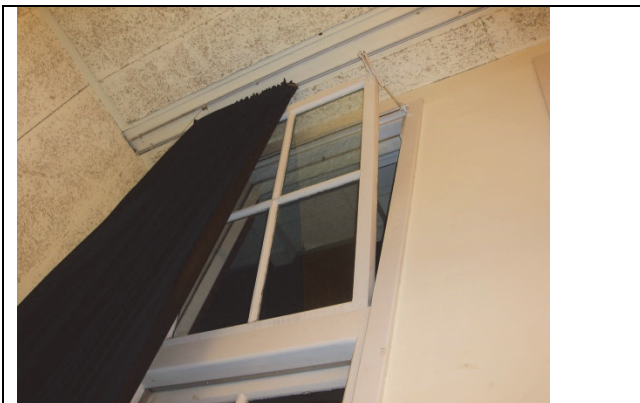
Figure 3.1.3: Bottom-hung window of a school in Poeldijk from 1921.
