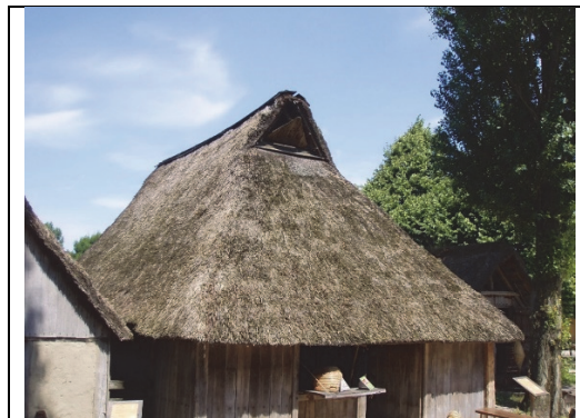
Figure 3.1.2: Example of a house of the early Middle Ages. The air exhaust can be controlled. The main original function of high openings was smoke removal, which has, without a chimney, a low effectiveness. When chimneys were being used air indoor quality and fire safety improved. (Archeon)
