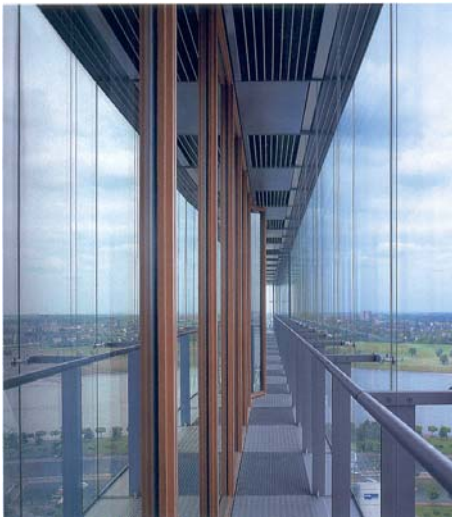
Figure 13: Double skin façade of the Stadttor in Düsseldorf 1997, designed by Petzinka (source: [1])
