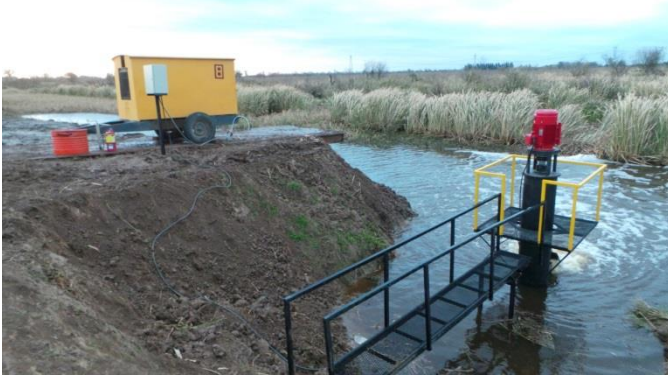
FIGURE 4 PICTURE OF A FORESTRY DYKE WITH PUMP
