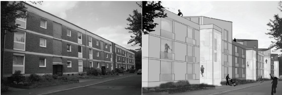
Fig.3. The existing front façade of the three- storey apartment block (a) and impression after the refurbishment (b).
