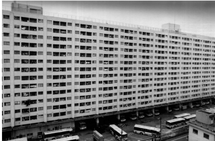
Figure 1 Bus terminal + housing. (from Made in Tokyo by Atelier Bow Wow, 2001)
