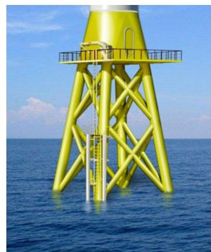
Figure 7.6: A schematic representation of a K-joint and how that would be applied in a jacket type foundation. [[100] & offshorewind.biz]
