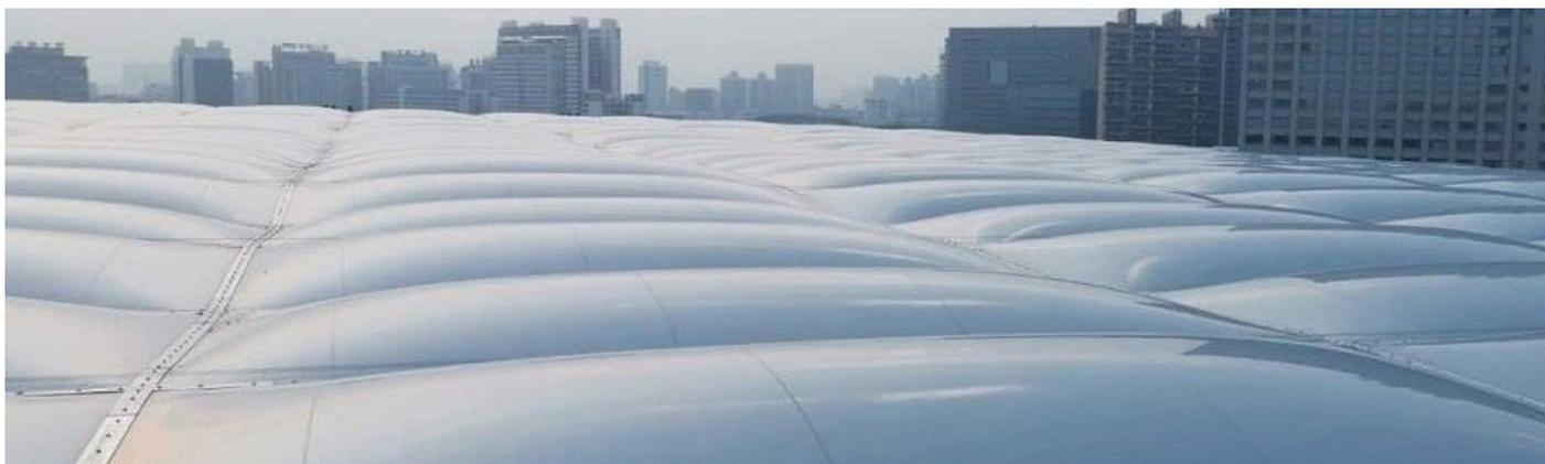
Figure. 14: Example of roof out of ETFE cushion panels (wikipedia)
