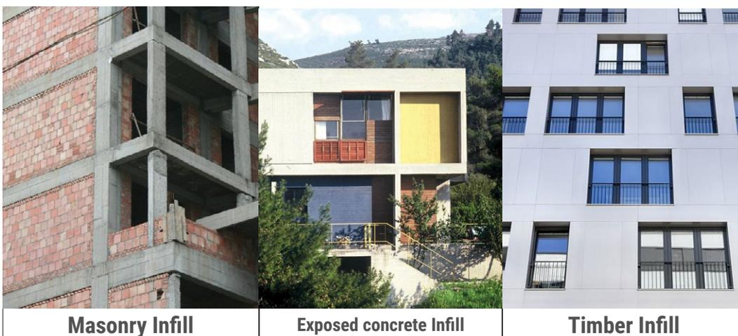
Figure. 9: Separation of facade systems based on material and structural aspects (Bianchi et al., 2024b)
