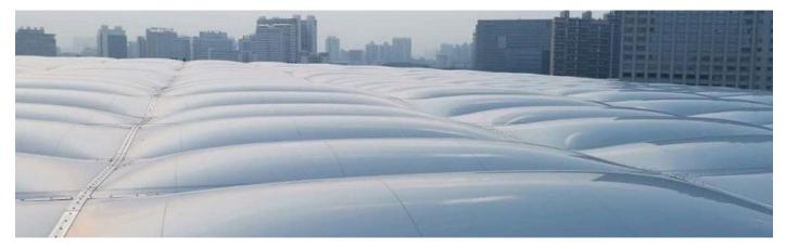
Figure. 14: Example of roof out of ETFE cushion panels (wikipedia)
