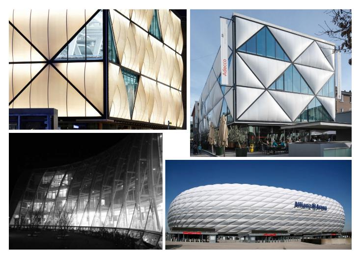
Figure. 15: Example of ETFE systems in buildings, Miroiterie Flon Lausanne at the top, Centre for Gerontology bottome left, Allianz-Arena bottom right
