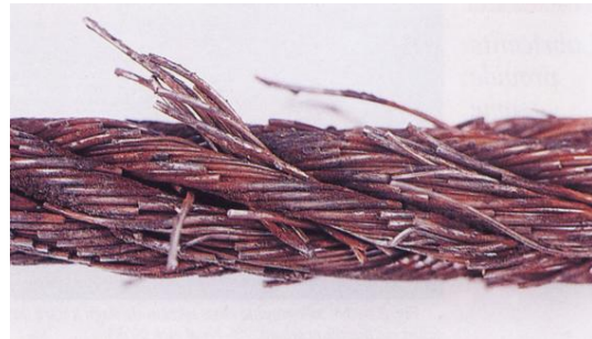
(b) Wire breakages as a result of rust.
