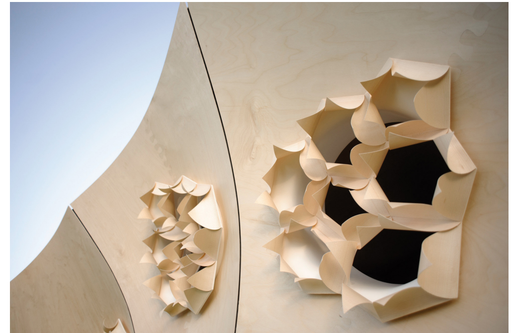
Figure 2.3 Wood lamellae in HygroSkin prototype. (Adsttc, 2023)
