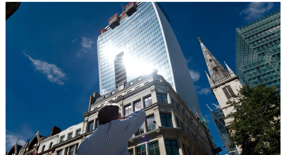
Figure 7.4 Curved glazing in a building that concentrates the solar radiation in a spot. The redirected radiation can increase the temperature and activate the SMA. (CNN, 2013)
