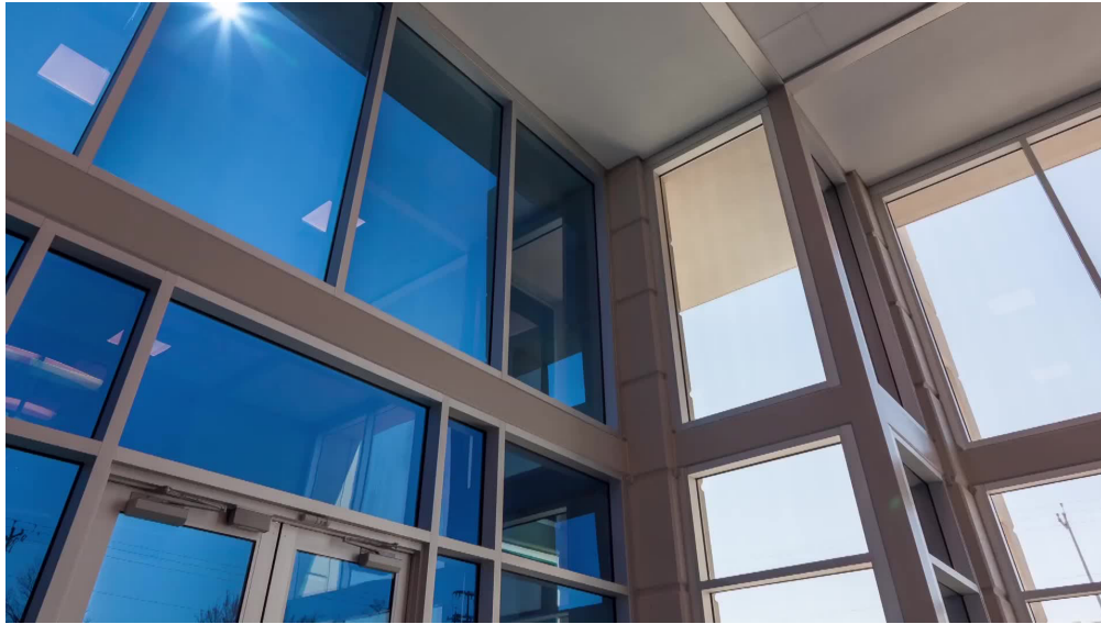
Figure 2.2 Active and inactive state of thermochromic glazing. (View, 2023)
