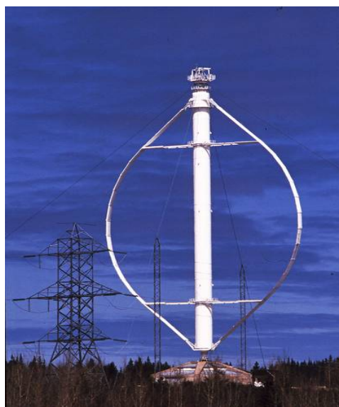
Figure 2.25: The Èole 4MW Darrieus VAWT (Gipe, 2016)
