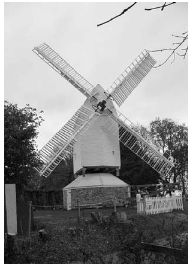
Figure 1.2: A north European wind mill also known as post mill (Manwell et al. , 2009)
