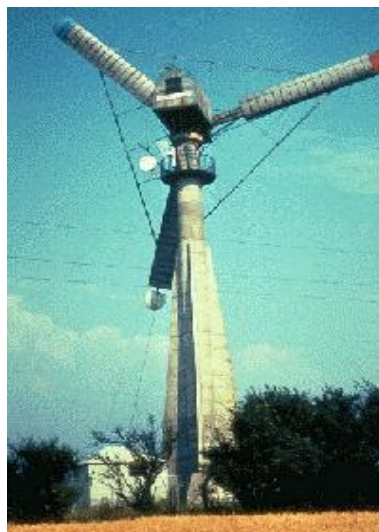
Figure 1.4: Gedser wind turbine (TelnosNet web development, 2015)
