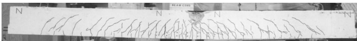
Figure 8.43 Crack pattern at failure load in experiment
