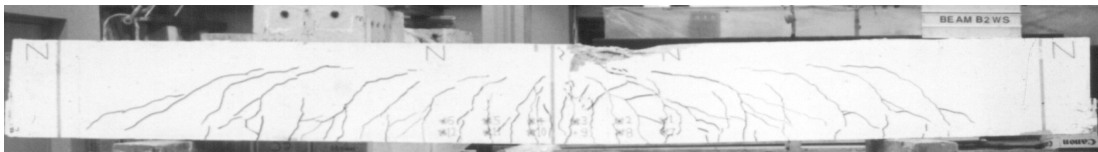
Figure 7.10 ULS crack pattern experiment B2 north face
