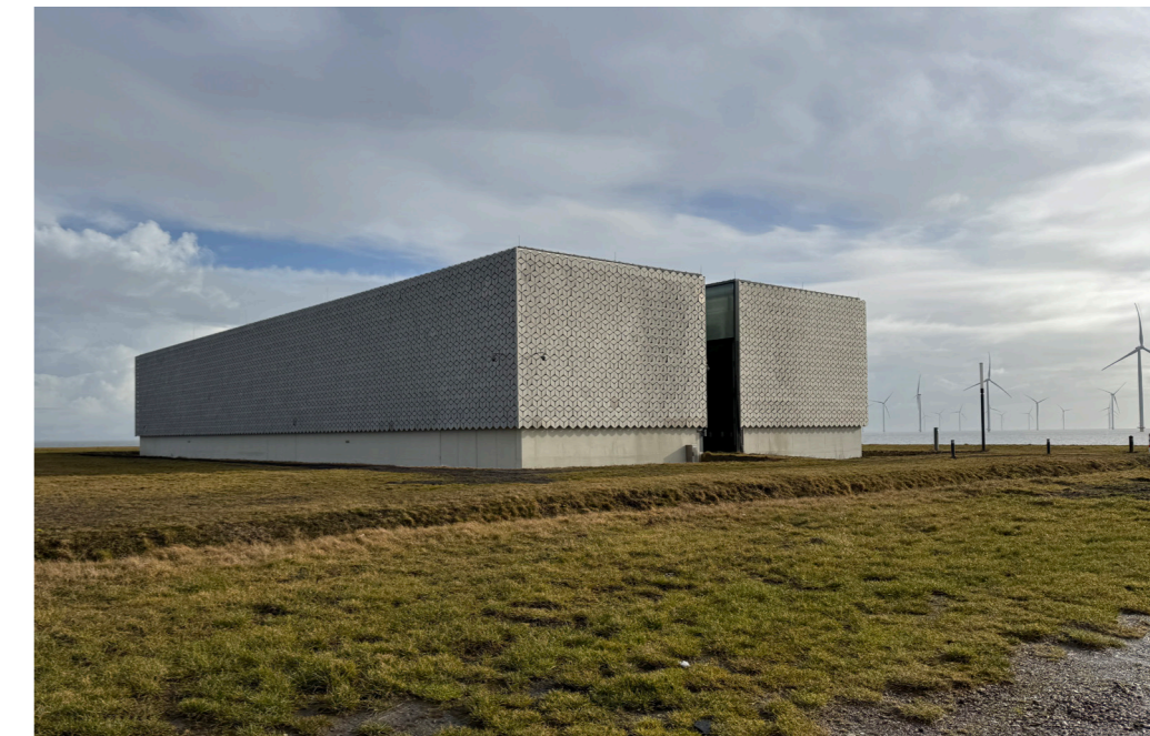
Figure 7.1: Breezanddijk Transformer Station at the Friesland (Fryslân) Wind Park
