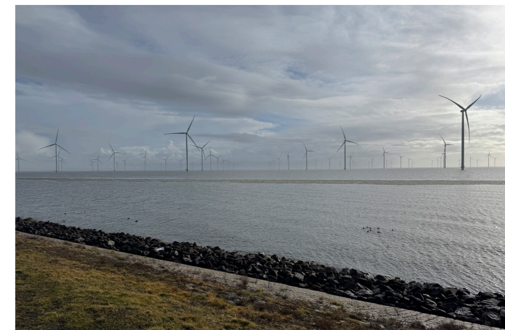
Figure 01: Frysland Wind Park in Friesland as seen from the Afsluitdijk
