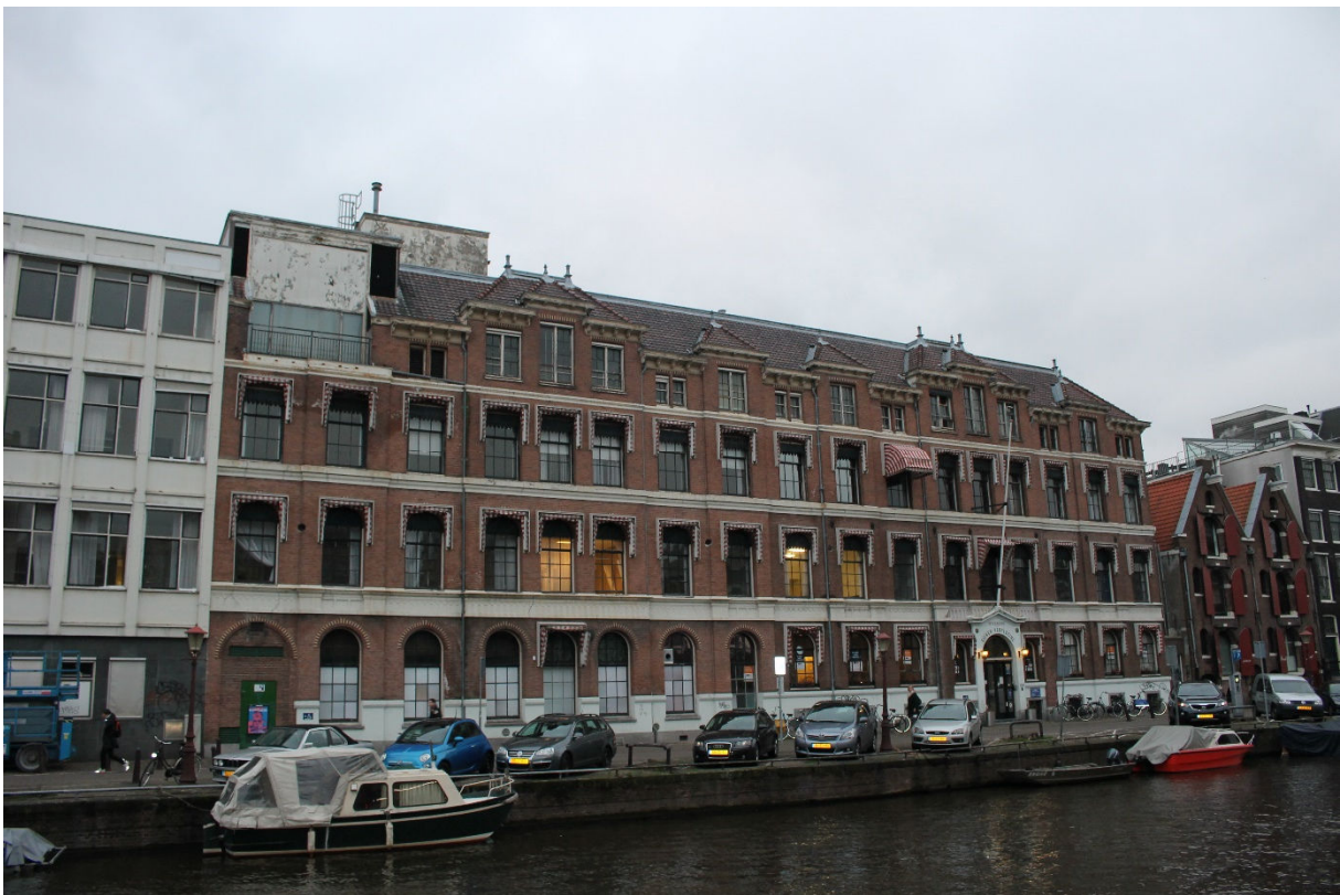
FIGURE 4.22 - TOP LEFT: STAIRWELL (CONCRETE). TOP RIGHT: ELEVATOR WITH ORIGINAL DOORS (?). BOTTOM: PRINSENGRACHT FACADE. THE 2ND AND 3RD FLOOR AND THE ROOF CONSTRUCTION DATE BACK TO THIS RENOVATION. PHOTOGRAPHS BY AUTHOR, 25-3-2015.
