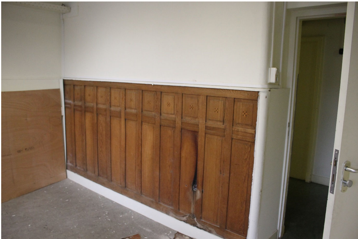
FIGURE 4.21 –WALL PANELLING BEHIND PRESSBOARD FACING. PHOTOGRAPH BY AUTHOR, 25-3-2015.
