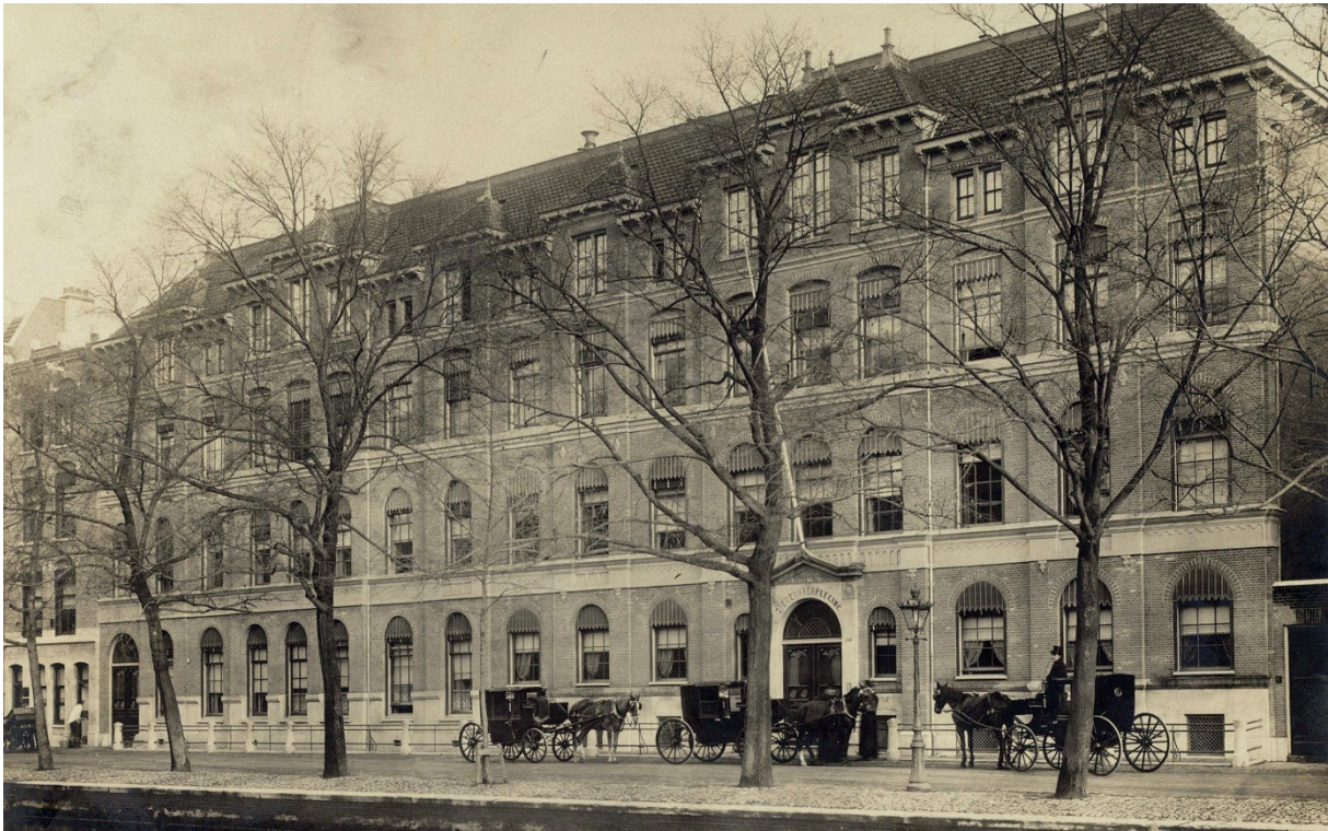
FIGURE 4.7 - THE PRINSENGRACHT HOSPITAL IN 1903. IMAGE: WWW.BIERMANHENKET.NL
