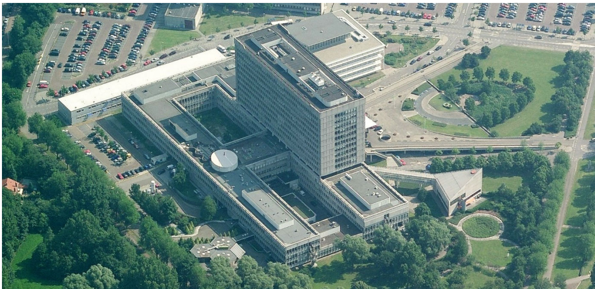
FIGURE 3.3 - THE LEYENBURG HOSPITAL IN THE HAGUE (ARCHITECTENBUREAU K.L. SIJMONS, 1971) IS AN EXAMPLE OF THE 'BREITFUß' MODEL. IMAGE: WWW.BING.COM/MAPS (ACCESSED 24-03-2015)
