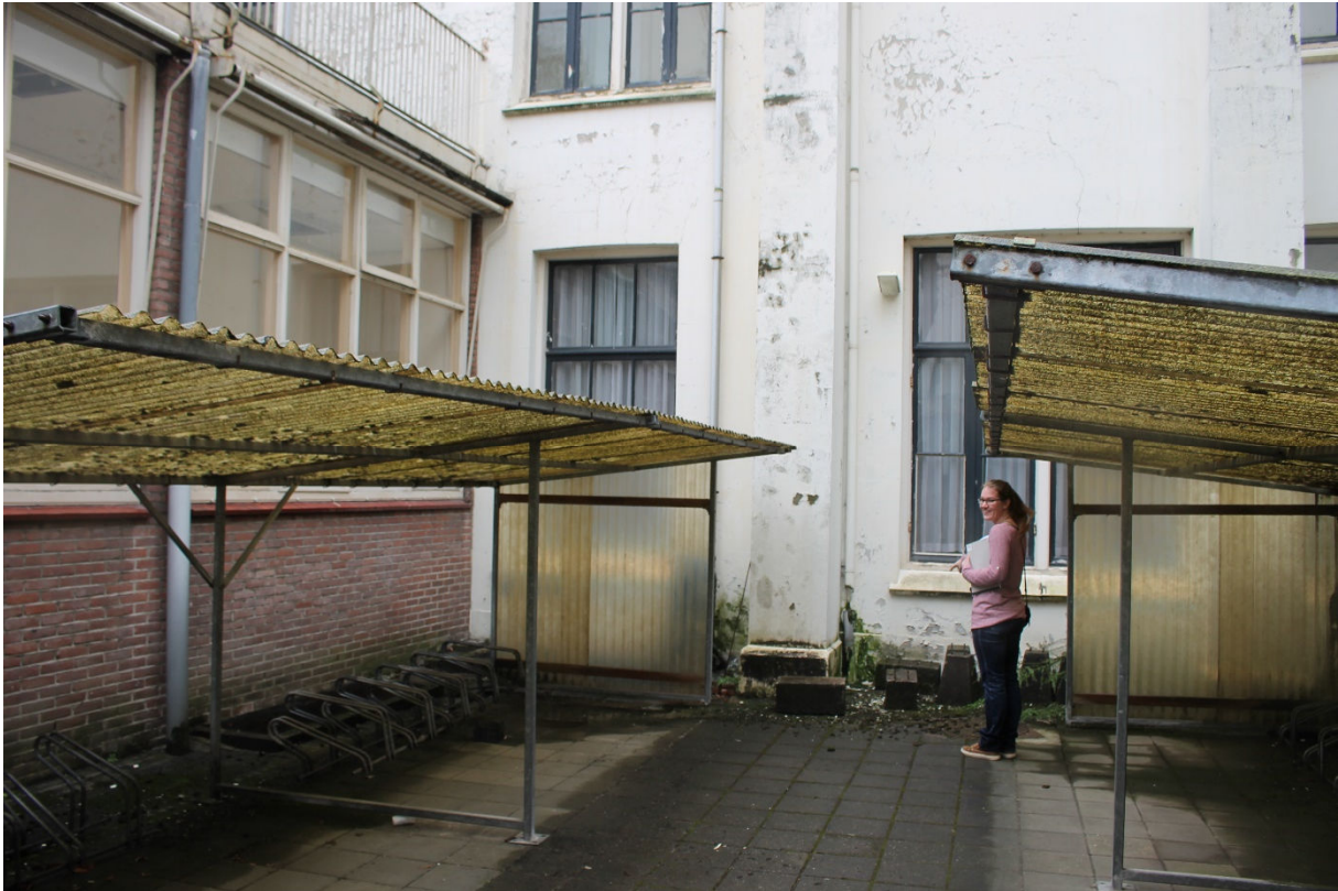
FIGURE 4.32 - VIEW IN THE COURTYARD. PHOTOGRAPH BY AUTHOR, 25-3-2015.
