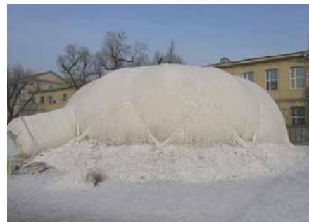
(b) Ice dome after construction.
