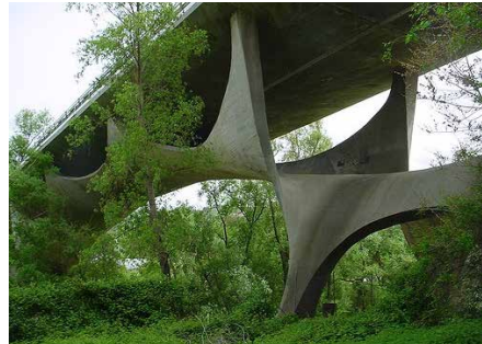
FIGURE 4.20 Figure 4.20: Basento Viaduct in Potenza, Italy, 1974 [108].
