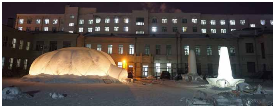
FIGURE 0.5 Three ice composite shells built at HIT, 2016
