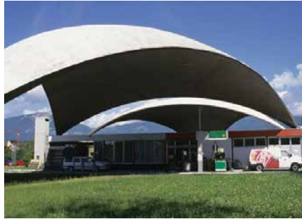
FIGURE 4.17 Deitingen Service Station, Switzerland, 1968 [104].
