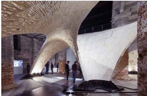
FIGURE 8.7 Tile vault prototype at ETH Zurich [151].
