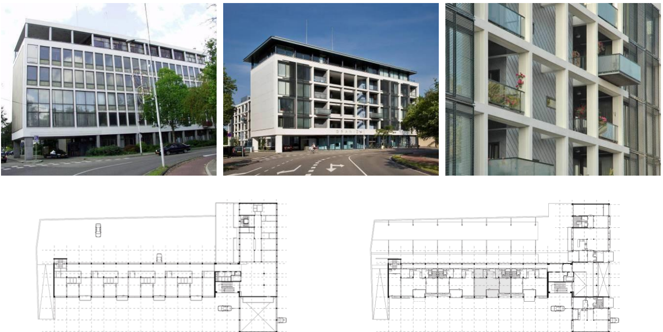
Figure 3: Granida. Left: the building before conversion; right: the building after conversion. The location near the city centre and the image of the building were important success-factors for this conversion. Alterations of the façade and a bad technical state of the structure led to high construction costs.
