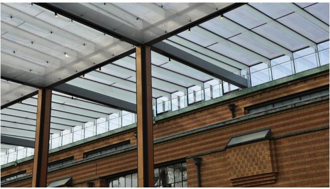
Fig 32. Newly designed extension of the roof over the courtyard with diffused natural lighting and coherence in materiality in Gemeentemuseum in the Hague, Image by author 2022
