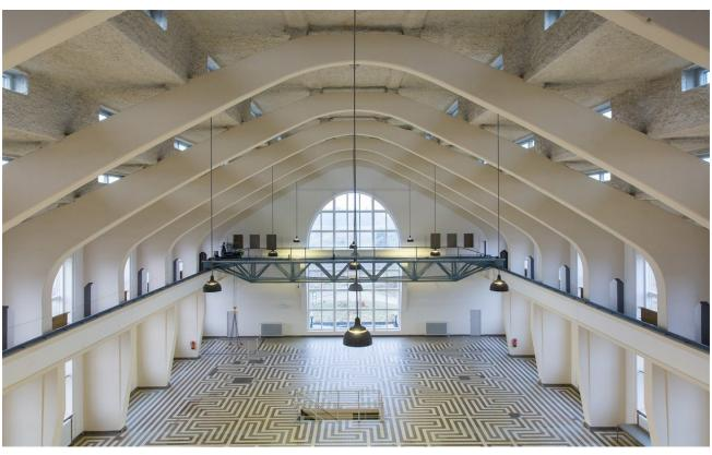
Fig 37. Heavy and repetitious concrete trusses in contrast with refined art-deco decorations and spaciousness in Radio Kootwijk in Apeldoorn, Staatsbosbeheer 2018
