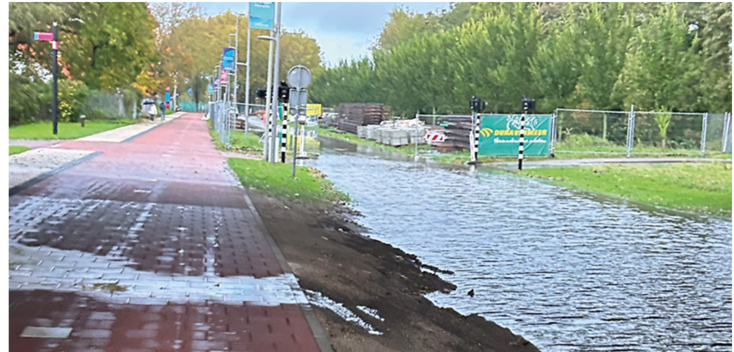
Figure: Photograph Mekelweg TU Delft Campus
