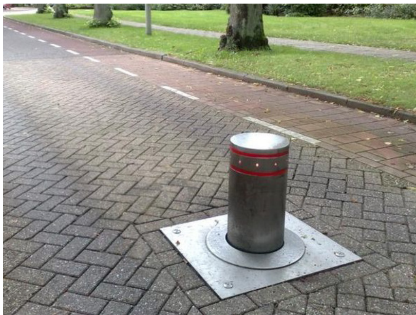
figure D.10 Traffic pole that can move up and down
