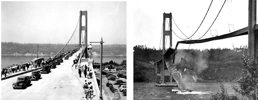
(a) The opening day of the Tacoma Narrows bridge at July 1, 1940 (University of Washington, 1940a). (b) The collapse of the Tacoma Narrows bridge at November 7, 1940 (University of Washington, 1940b).
