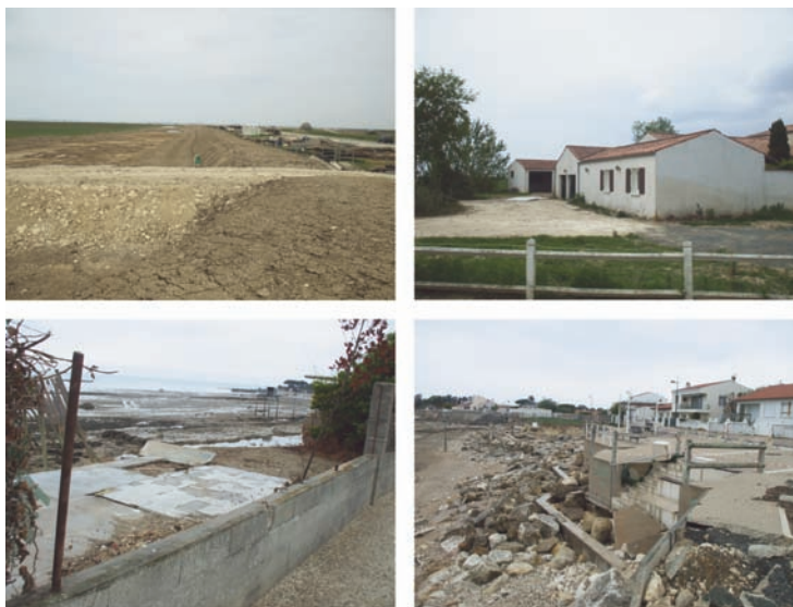
Figure 24: Clockwise: emergency dike in Charron, house in Charron showing that the water level rose to 1.5 m, destroyed promenade of Chay near Chatillon Plage, destroyed house near the coast only the kitchen floor is still visible.
