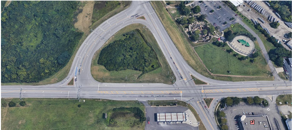
Figure 5 State Route 4 at State Route 4 Bypass/Ross Road, Fairfield, Ohio.
