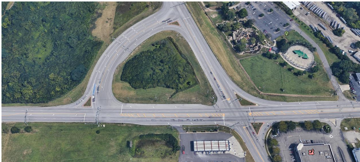
Figure 68 State Route 4 at State Route 4 Bypass/Ross Road, Fairfield, Ohio.
