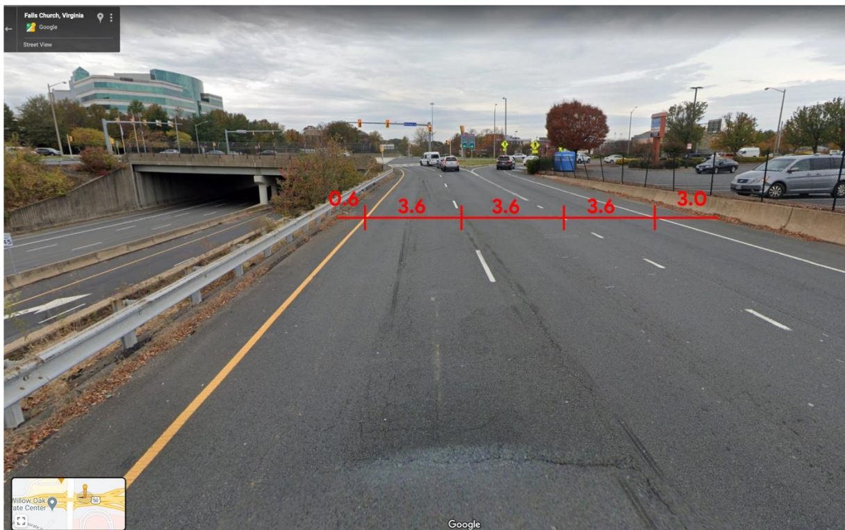
Figure 3 Dimensions of road 2 that does not comply with the Dutch guidelines.
