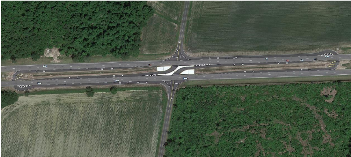
Figure 70 Highway 9 East at Liberty Church Road, Loris, S.C.
