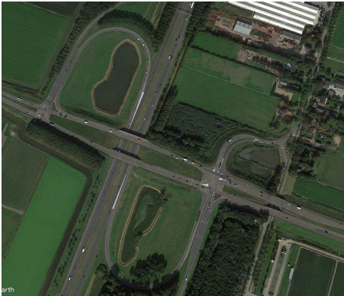
Figure 15 Location 2 Parclo interchange.
