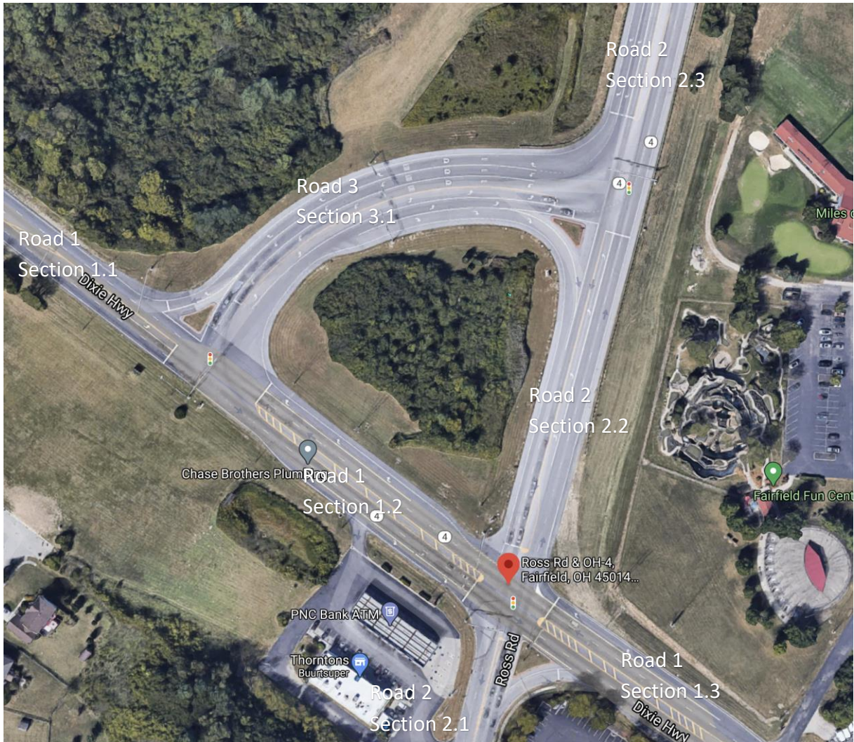
Figure 80 State Route 4 at State Route 4 Bypass/Ross Road, Fairfield, Ohio.
