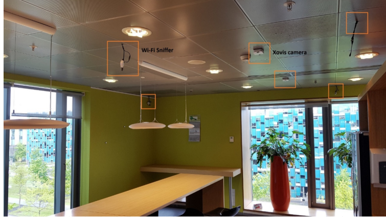
Figure 4.13: Wi-Fi sniffers and cameras deployed in the coffee corner area
