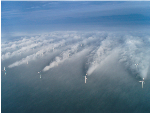
Fig. 6. Horns Rev offshore wind farm with, normally invisible, wakes. Source: Christian Steiness. See also [30] for more information on the picture.
