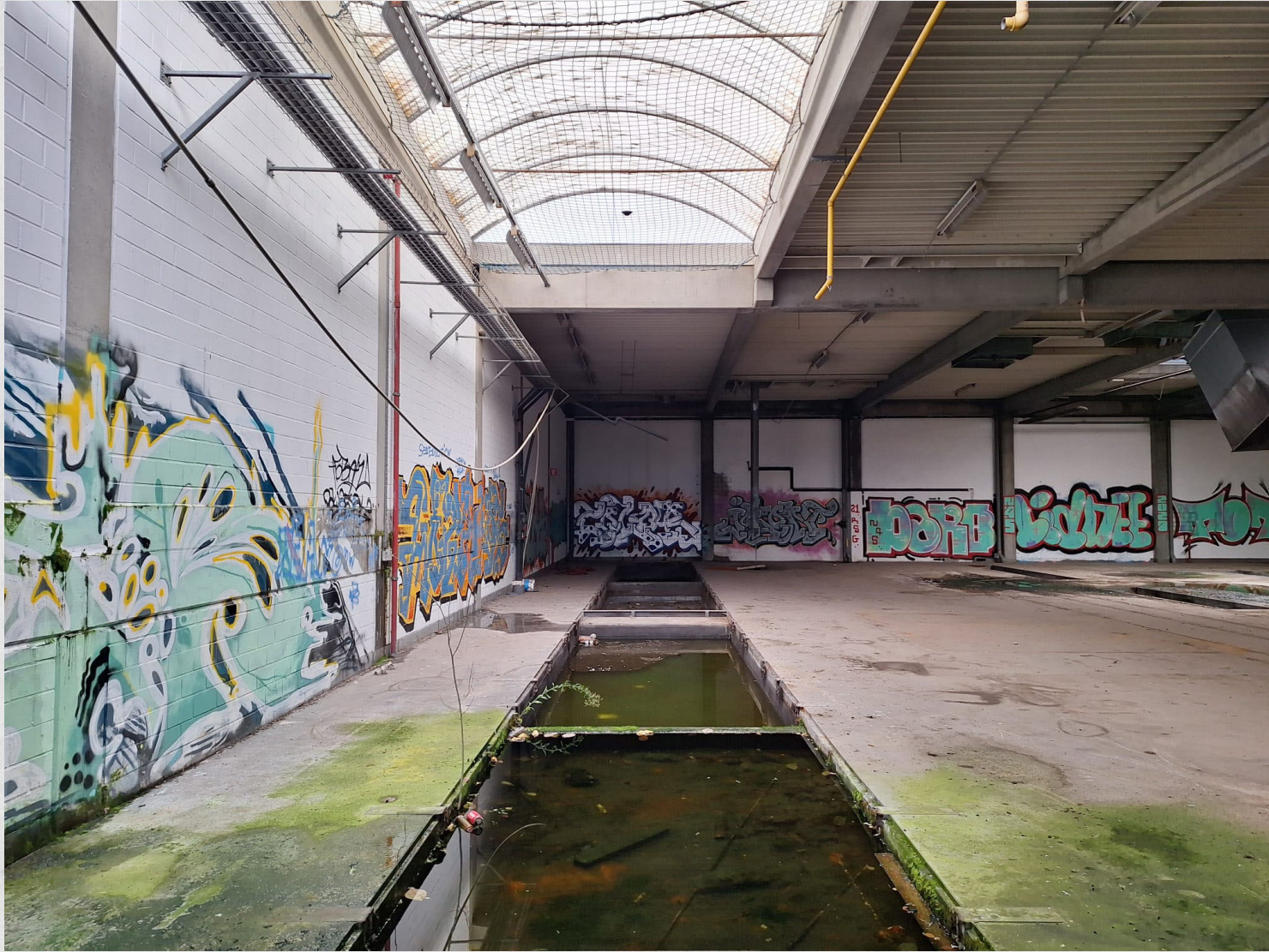
Photo of the concrete hall with a light steel roof and large roof lights; and existing prefab gutters.
