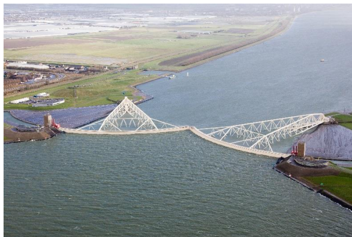
Figure 1 Maeslant barrier in closed position (Rijkswaterstaat)
