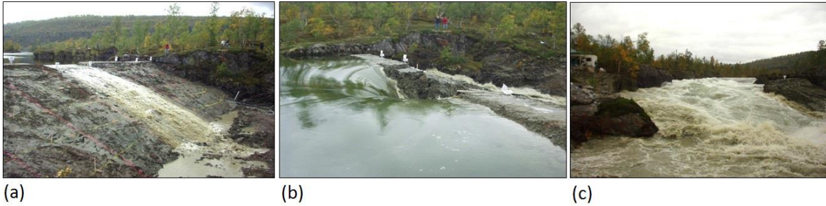
Figure 1: flow profiles over an embankment during erosion.
