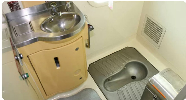
Figure 27. Chinese style toilet
