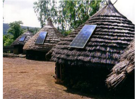
Figure 1.4: Thatched roof houses aligned with PV panels as part of Solar Home Systems (SHS) in African rural areas [18]
