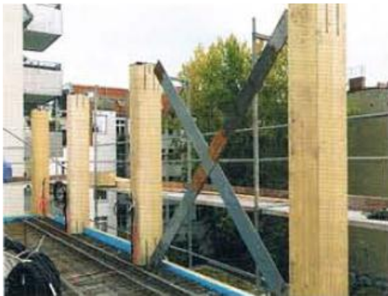
figure A.1: Pictures of bracing [32]
