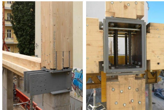
figure A.2: Pictures of connection details [32]
