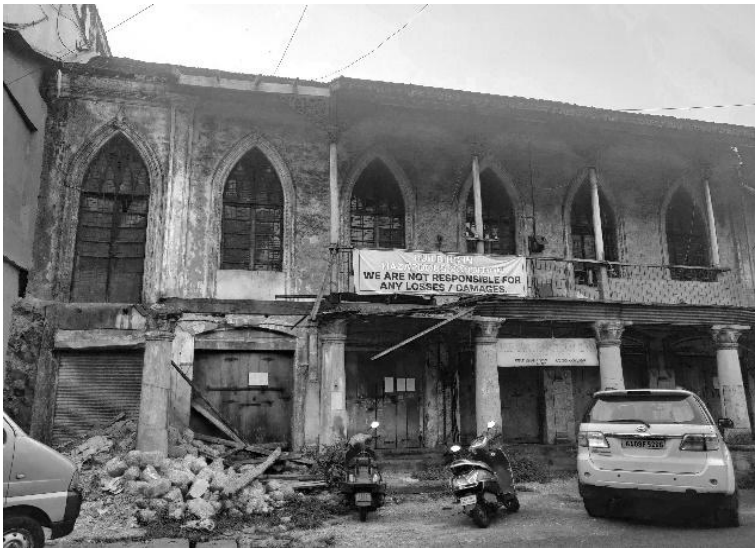
Figure 62: House on Rua Abade Faria in a dilapidated state
