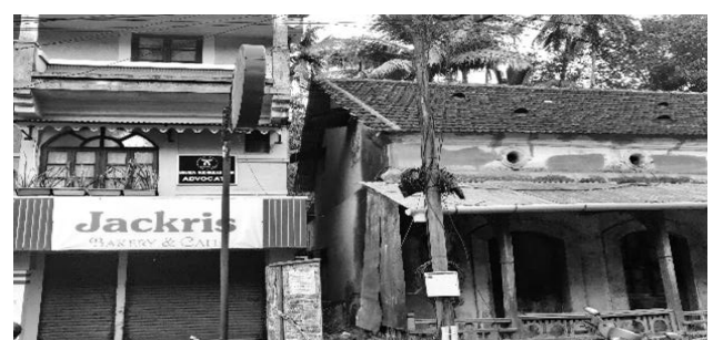
Figure 12: Modern material inserts within an existing structure
