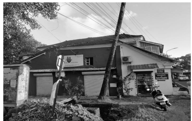
Figure 10: Modern material inserts within an existing structure
