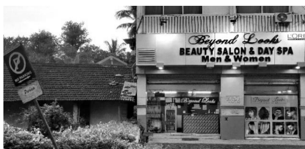
Figure 11: Modern material inserts within an existing structure
