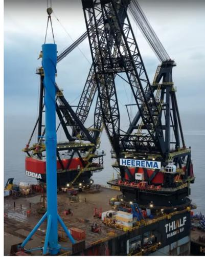
**Fig. 2-2 In-situ installation of the tower with C1 wedge connection [1]**
