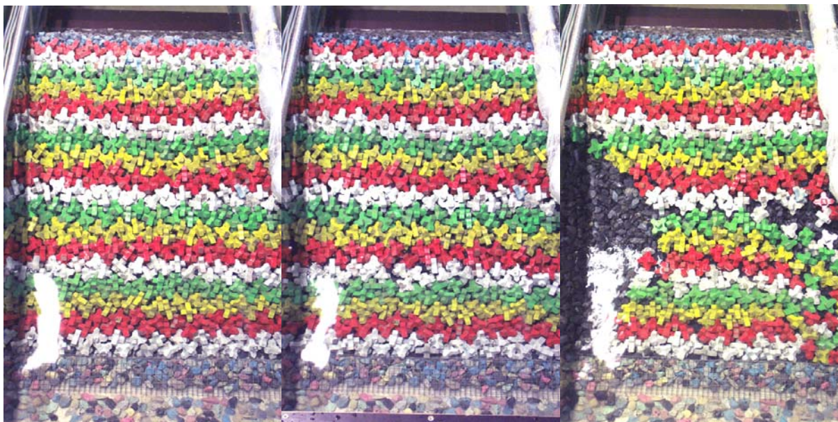
Picture 3-5: Damage to the Xbloc layers
