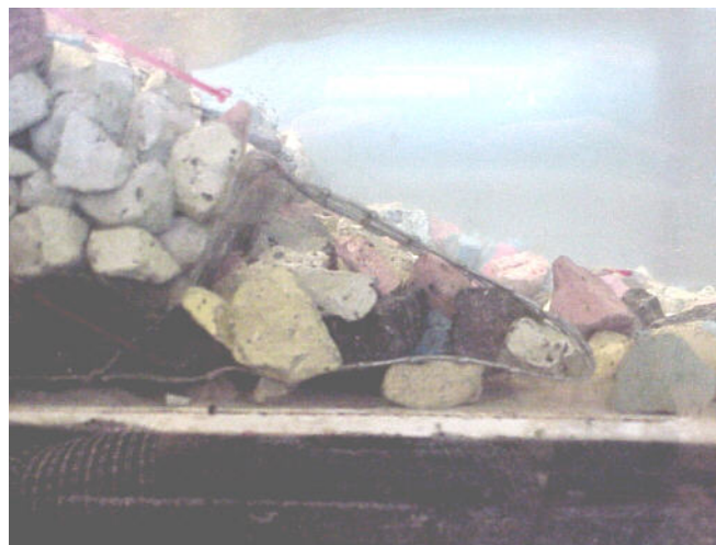
Picture 2-6: Detail of the toe
