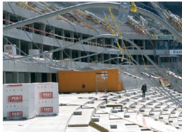
Figure 3.14 Erection of the cable ring structure [39].
