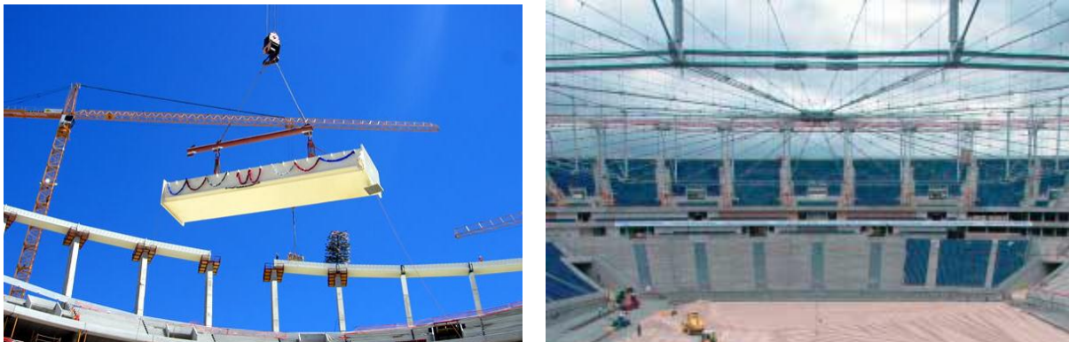
Figure 12.6 Construction concrete compression ring at Greenpoint stadium (left) and construction of cable net structure at the Commerzbank Arena (right)
