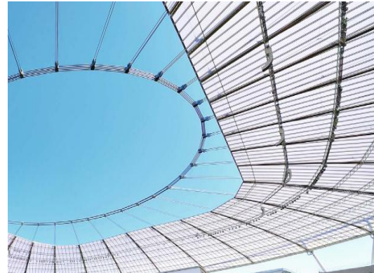
Figure 3.15 Aerial view BayArena, Leverkusen
