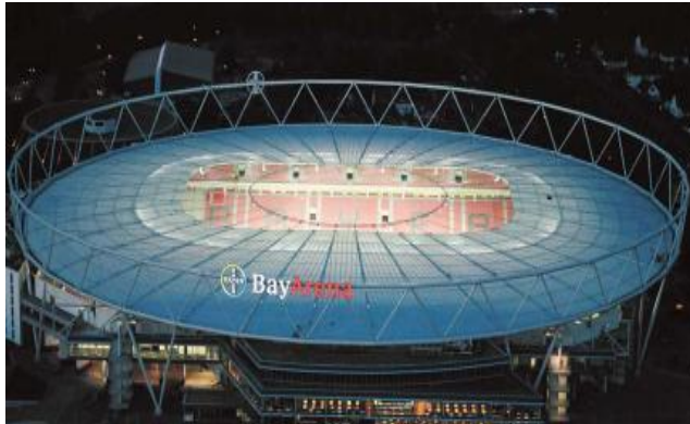
Figure 3.16 Aerial view BayArena, Leverkusen
