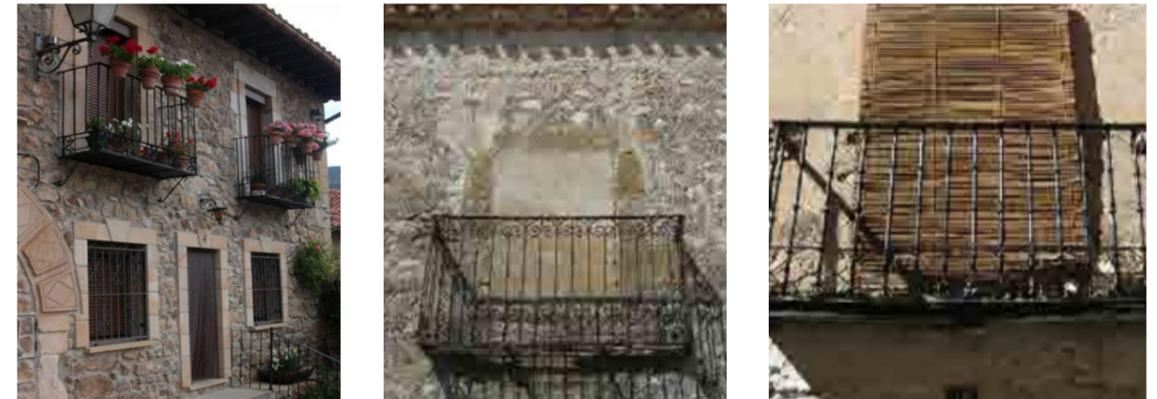
Fig. 88 Examples of railings, according to traditional steel balconies (Martinez, 2011; Moreno Dopazo, 2014).
