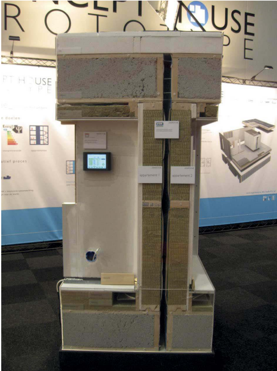
FIG. 67 Mock-up with apartment dividing wall [a.o.]
