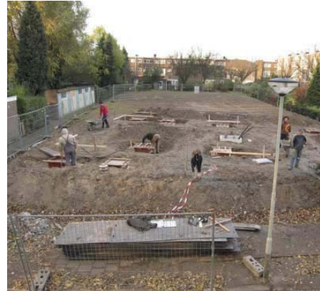
FIG. 85 Driving in the first pile (left), and laying the foundation in the conventional manner
