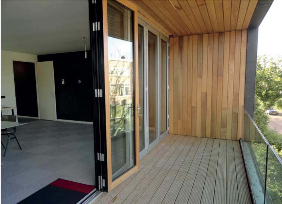
FIG. 73 Realised Solarlux folding facade
