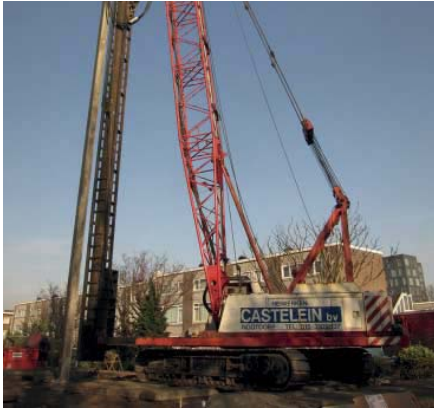
FIG. 85 Driving in the first pile (left), and laying the foundation in the conventional manner
