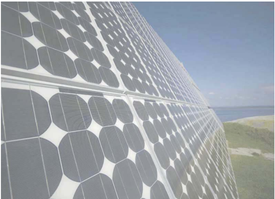
FIG. 44 Installation of PV cells to generate electricity
