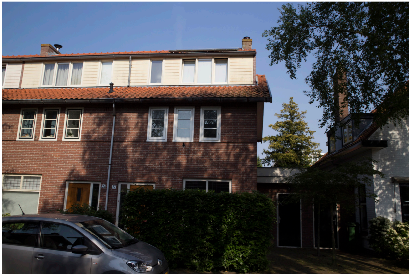
figure (32f) front view of typical existing added roof structure (source: own image)
