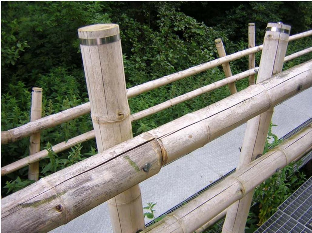
*Figure 20: Cracking of bamboo culm when directly exposed to climatic conditions*
