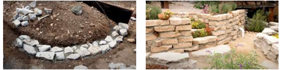
Figure 26 Retaining Wall ( https://www.youtube.com/watch?v=aM4FWHb75mE )
