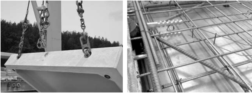
Figure 155 Lifting Of A Precast Wall By Embedded Anchor Points
