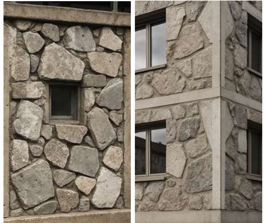
Figure 153 Thick Rubble vs Thin Rubble (AI & Collage)
