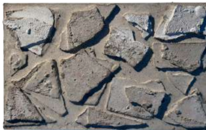
CS Rubble 2 Rough Surface
