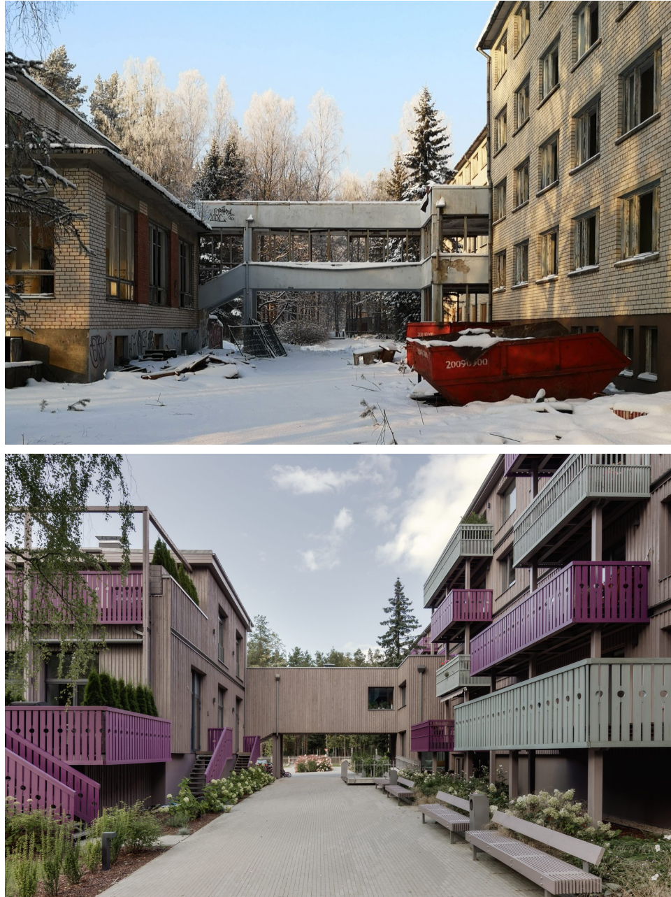
Fig. 3.3. Renovation of Edinburgh Apartments & Lofts in Jurmala, Latvia, by Open Architecture Design.
