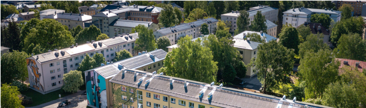
Fig. 2. 3. Khrushchevka renovation concept in the SmartEnCity project.
