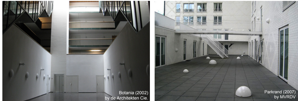
NON-FUNCTIONING COLLECTIVE SPACE
