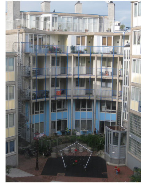
South-oriented courtyard facade
