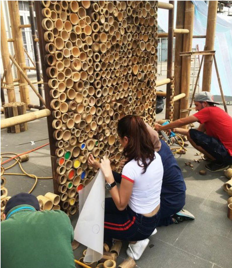
Pavilion by Eleena Jamil. Source: https://ej-architect.com/
