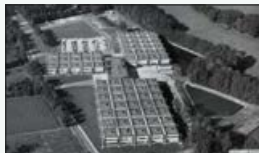
● 1964 All-purpose building 'De Hallen' S.J. van Embden / J. Choisy
